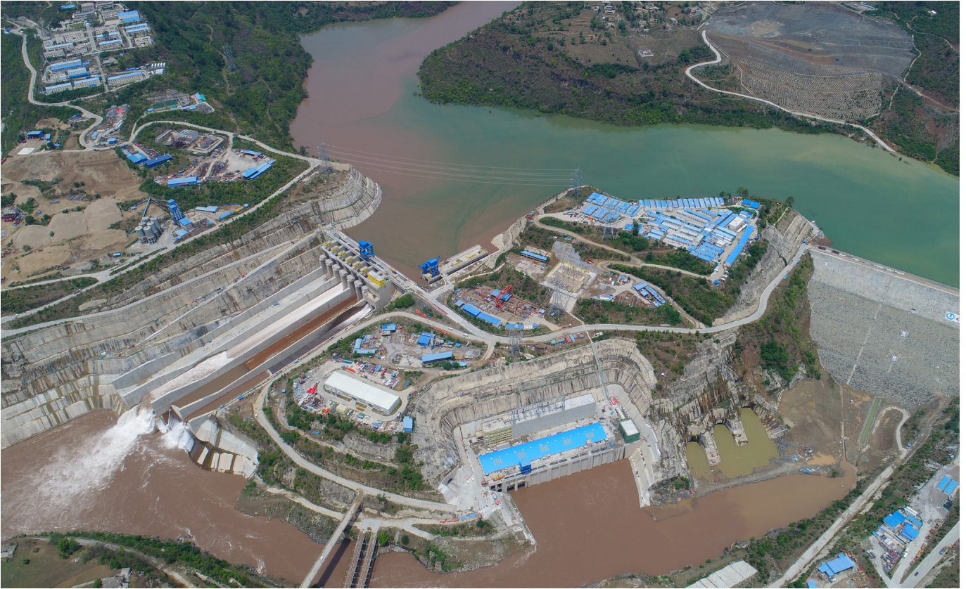
Aerial photo taken on June 22, 2022, shows a view of the Karot Hydropower Project in Punjab province, eastern Pakistan. (XINHUA)
