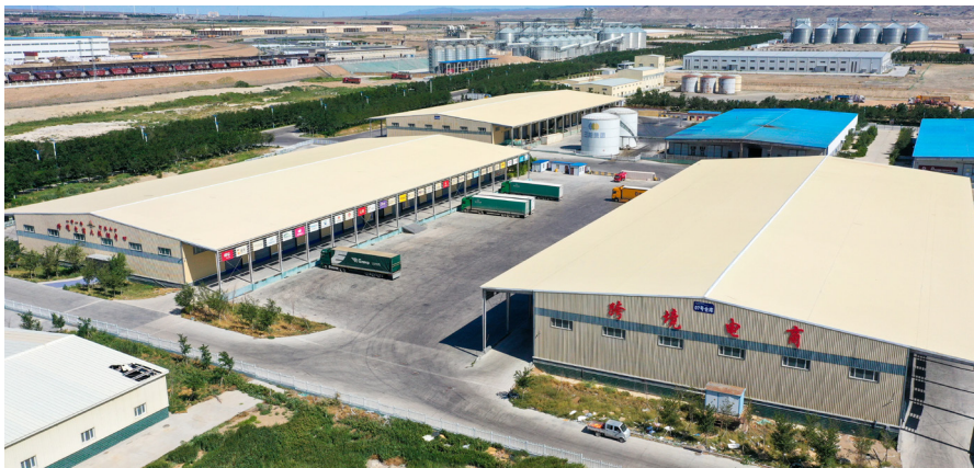
This aerial photo taken on July 24, 2023 shows the custom clearance center for the cross-border e-commerce of the Alataw Pass comprehensive bonded area in northwest China's Xinjiang Uygur Autonomous Region. In recent years, various measures have been taken to create a better business environment for cross-border e-commerce enterprises in Alataw Pass. (XINHUA)
